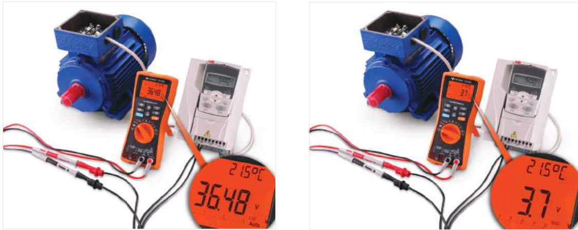
Figure 2. U1272A helps you identify the presence of stray voltage on a disconnected wire running parallel with the wire powering up the VFD to an industrial motor. The image on the right shows the U1272A in low impedance mode.
